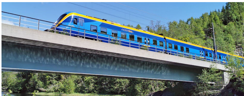
Figure 2: The bridge with a long-term monitoring system.
