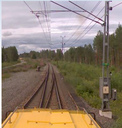
Cant compensation due to curve
