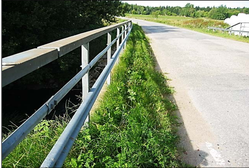
Figure 1.6: Vegetation growth that subsequently aids biological attacks on the BEBS Source: Johan Silfwerbrand
